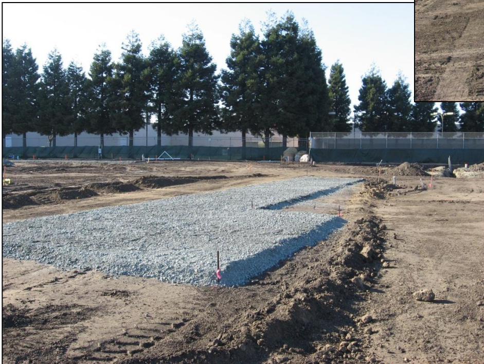
SLUSD Pacific Sports Complex & Burrell Field: Dugout foundation at baseball fields
