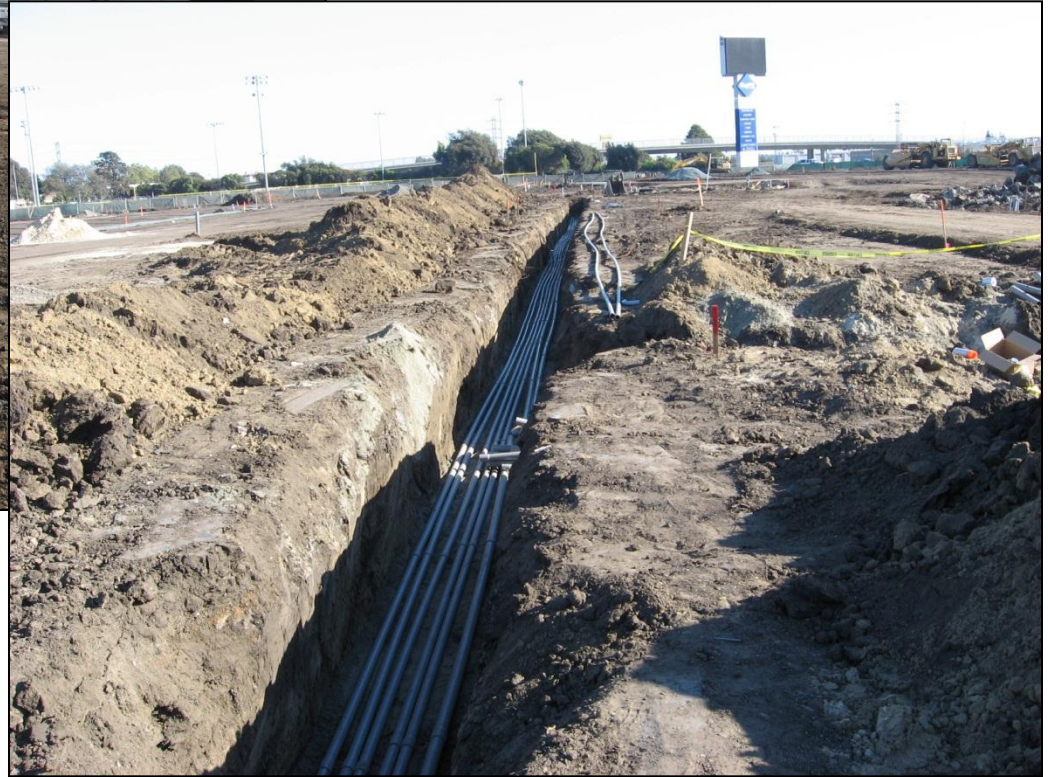
SLUSD Pacific Sports Complex & Burrell Field: Drainage and underground utility
