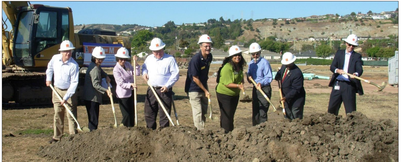
SLHS Swim Center, Track & Field Groundbreaking on August 30, 2012
