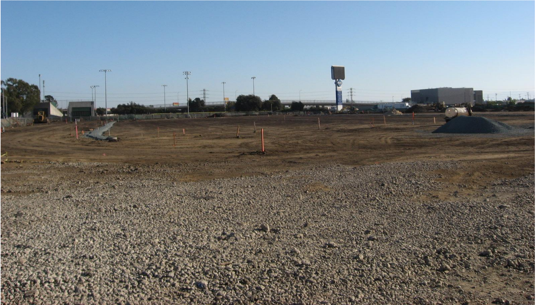
SLUSD Pacific Sports Complex & Burrell Field: grading of football field
